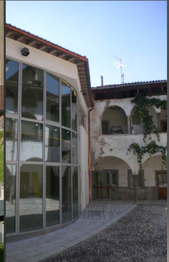
Refurbishment of ex Convent – Fino del Monte (BG) - ITALY
