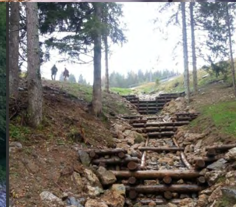
Hydraulic engineering works - Valgoglio (BG) - ITALY
