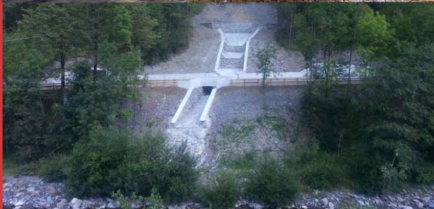
Hydraulic engineering works - Valbondione (BG) - ITALY
